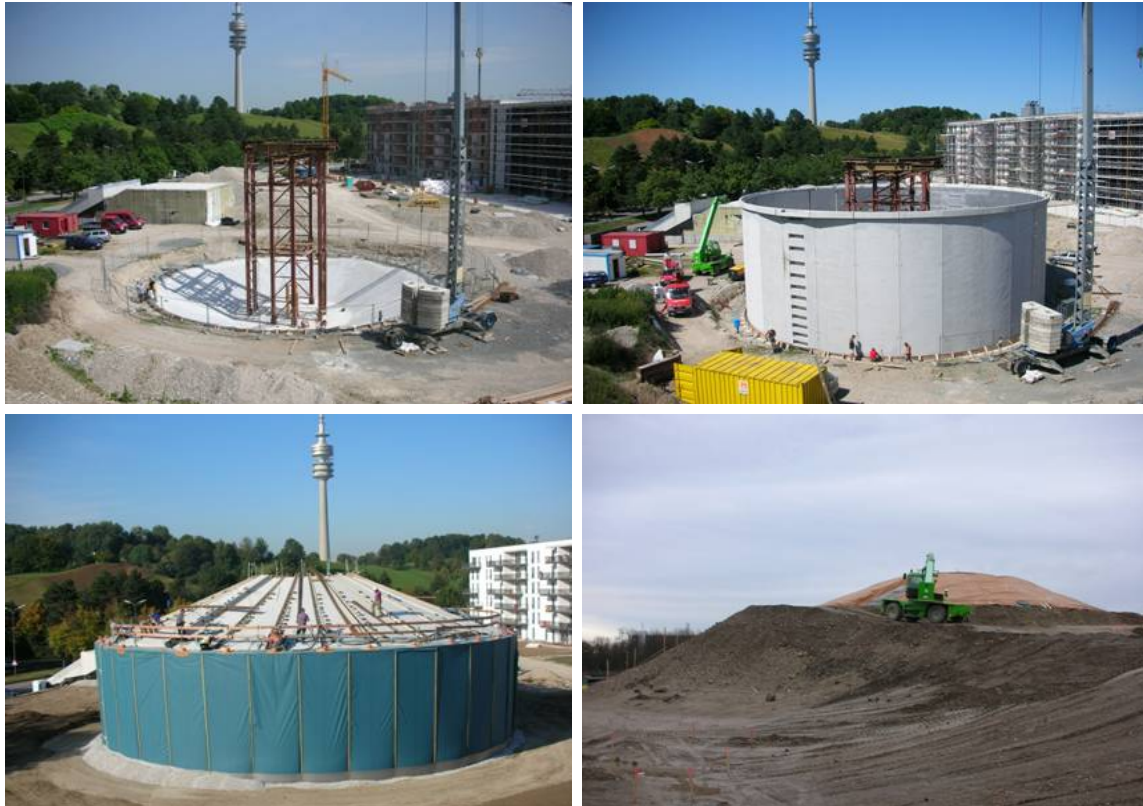
Fig. 3: Construction of the tank thermal energy storage in Munich, 2006.
