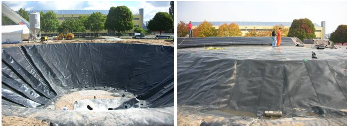
Fig. 4: Construction of the pit thermal energy storage in Eggenstein, 2007.
