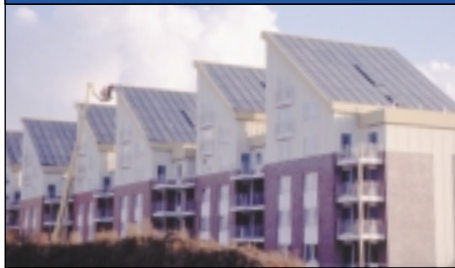
Fig 8: 1000 m 2 Solar Roof; North-south multi-family dwelling (Rostock)
